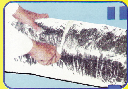
1 Cut jacket fiberglass and inner care with knife.
