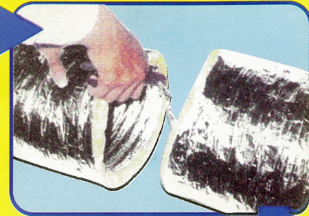
2 Cut noise of inner care with pliers.
