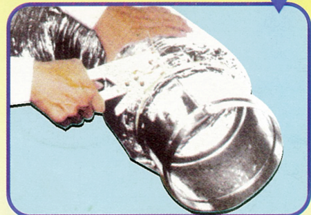
4 Put insulation and jacket over taped inner care and clamp.
