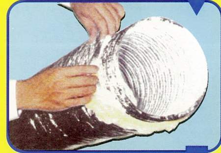
3 Pull back fiberglass insulation leaving outer jacket.
