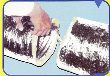
2 Cut noise of inner care with pliers.
